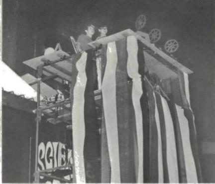
Ten slide projectors, three 16mm motion picture projectors, two operators and one spotlight with color wheel were jammed atop the 18-foot scaffolding to provide the six-screen visual effects for 1968
